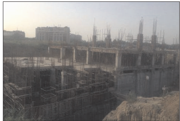
Construction of Surgical Block, AIIMS, New Delhi
