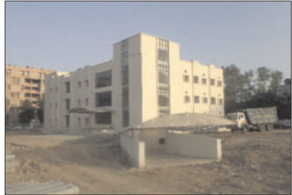
Construction of Dining Block, AIIMS, New Delhi
