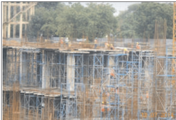
Construction of Super Speciality Block, Safdarjung Hospital, New Delhi
