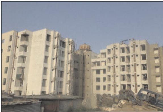
Construction of Hostels at AIIMS, New Delhi
