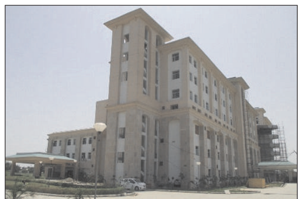
Construction of All India Institute of Ayurveda
