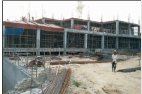
Construction of Kalpana Chawla Govt. Medical College, Karnal
