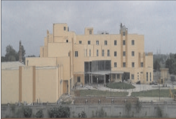
Construction of 100 bed Advanced Cancer Diagnostic Treatment & Research Centre, Bhatinda
