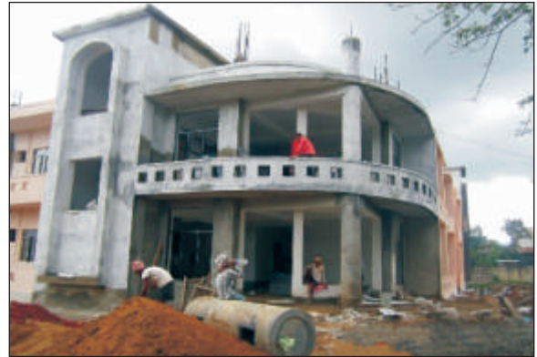
Construction of Hostels for Regional Institute of Medical Sciences (RIMS), Imphal
