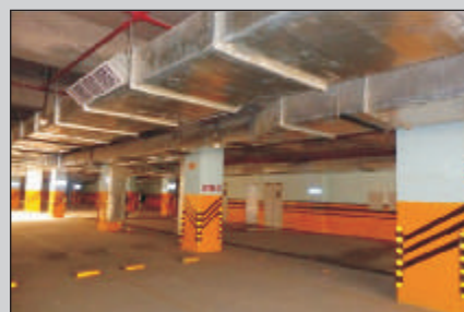
AIIMS - Under Ground Parking New Delhi
